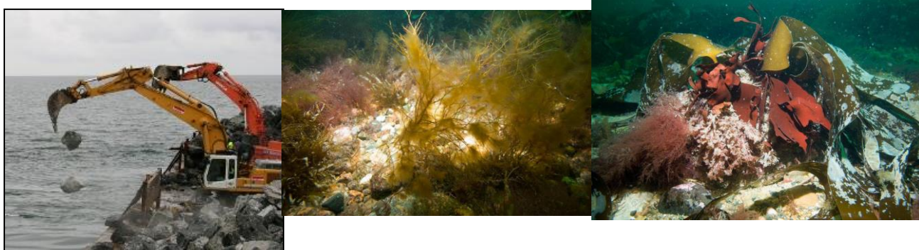
Fig. 15 - Laeso Trindel artificial reef: construction of the reef (left) and benthic colonization on the reef boulders (from Dahl et al., 2009).
